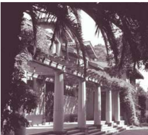
Gone but not forgotten: Julia Morgan designed the gymnasium above, along with Alumnae Hall and Hellman Pool, to form a U-shaped complex on the edge of Toyon Meadow. Only Alumnae Hall, now known as the Student Union, still stands.
